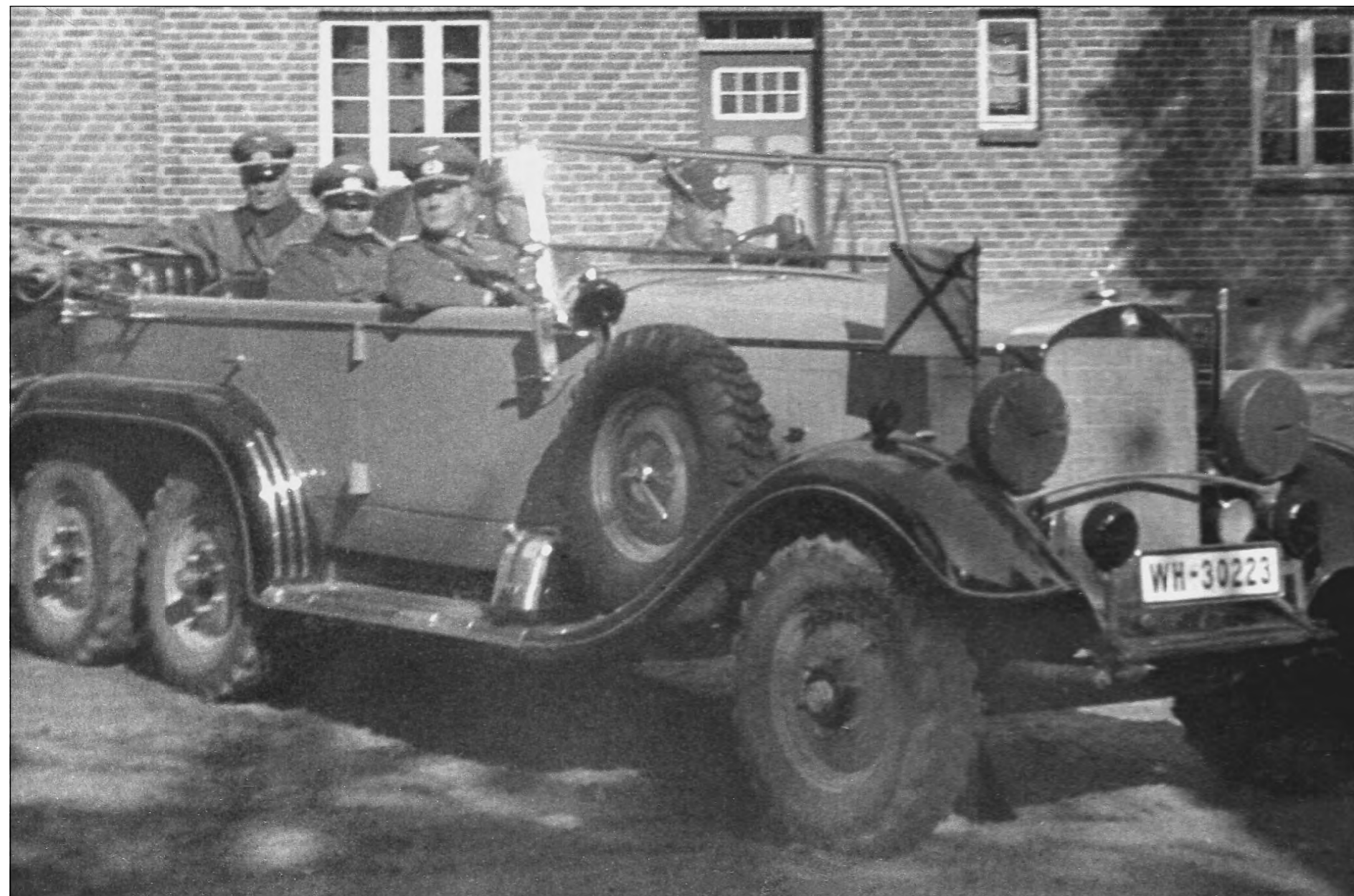
In this photograph, Generalfeldmarschall Werner von Blomberg rides in one of the earliest versions of the G4. The difference in the rear wheel arch with regard to the G4-540 is clearly visible. The spare fuel can stowed on the right side of the Mercedes is also totally different to subsequent models. (K. Miller Collection).
